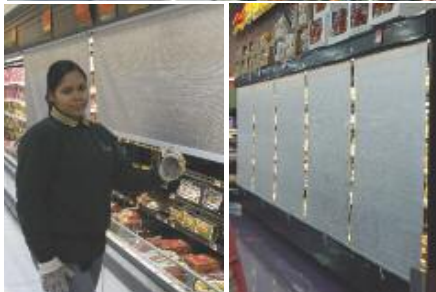
Econofrost's night covers are available with centralized controls for automated operations or manual pull-down covers.
